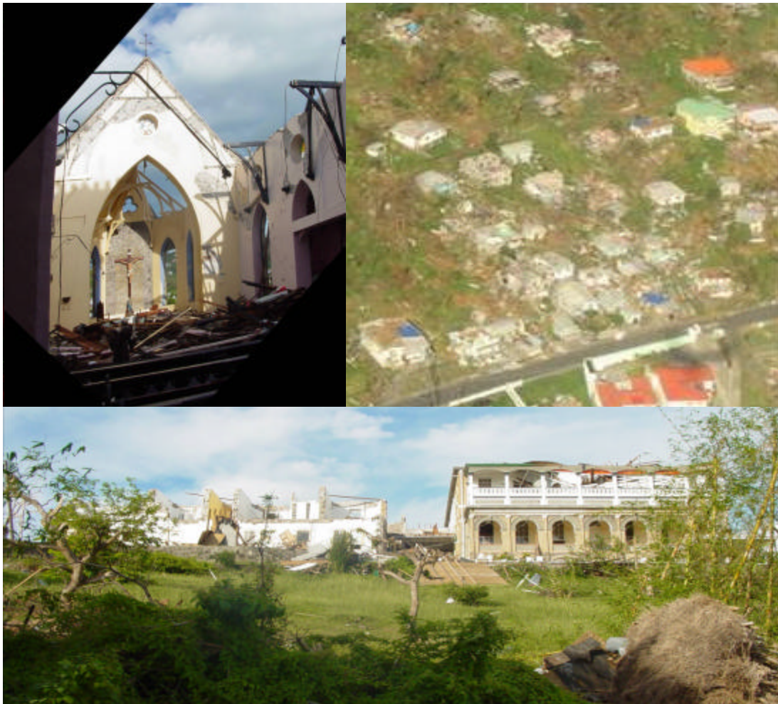
Figures 10–12. Hurricane Ivan destruction
