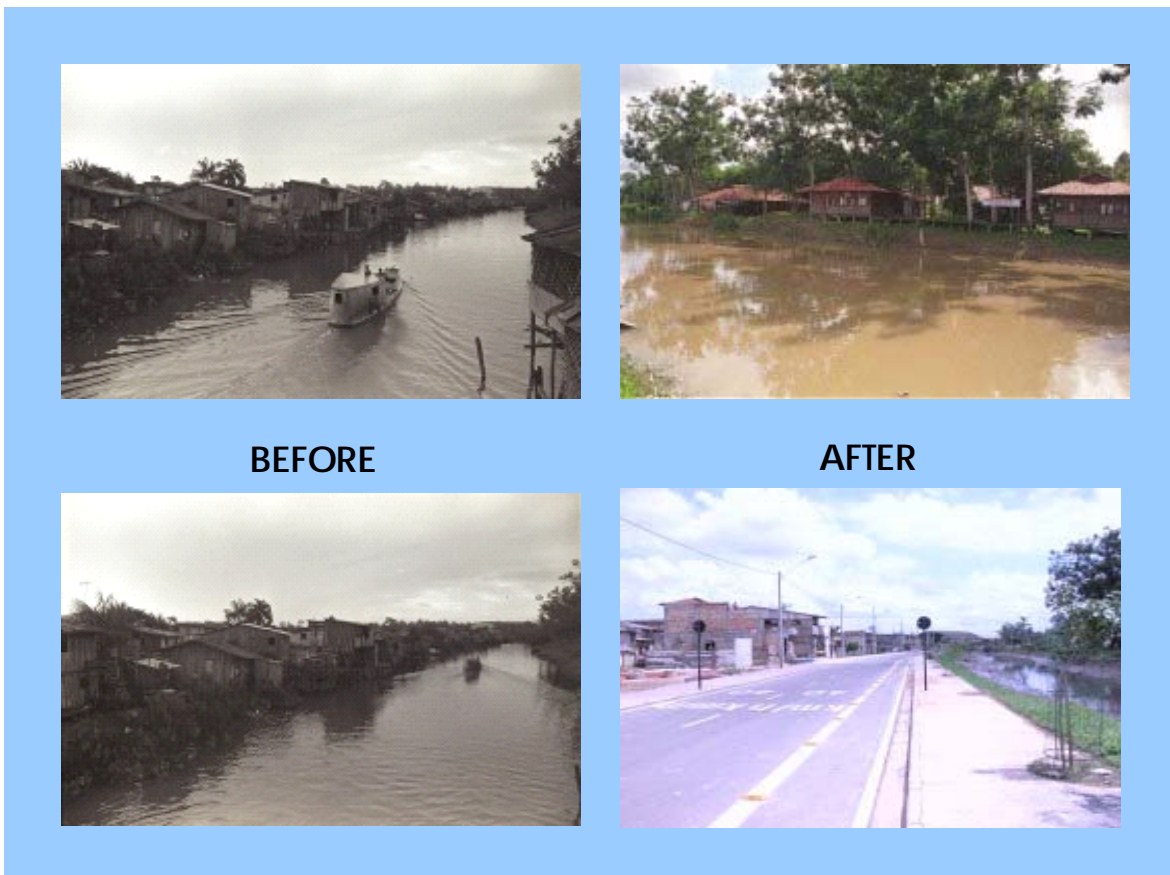
Figure 6. Canal-draining project: Tucunduba Basin
