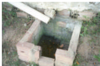
.Open drainage box for household wastewater is "open house " for Culex quinquefasciatus mosquito breeding. However this box can be sealed against mosquitoes. Photo courtesy of Steven Ault, 2003.
