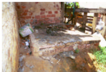
Abandoned and/or unimproved pit latrines are ideal breeding sites for Culex quinquefasciatus , and should be filled up with dirt and replaced with VIP latrines or sanitary sewerage. Photo by Steven Ault, 2003.
