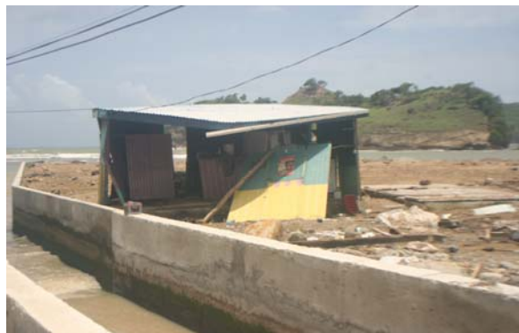
Photo 4 – Damaged property at Dennery
