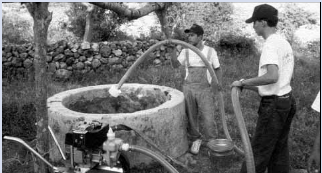
Nicaraguan workers clean a water well contaminated during Hurricane Mitch in 1998. Such efforts prevented any major outbreaks of cholera.
