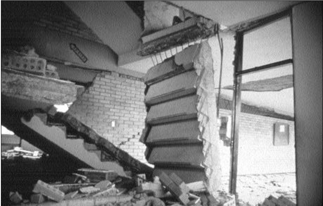
Photograph 6. Collapse of stairway during earthquake prevents evacuation.
