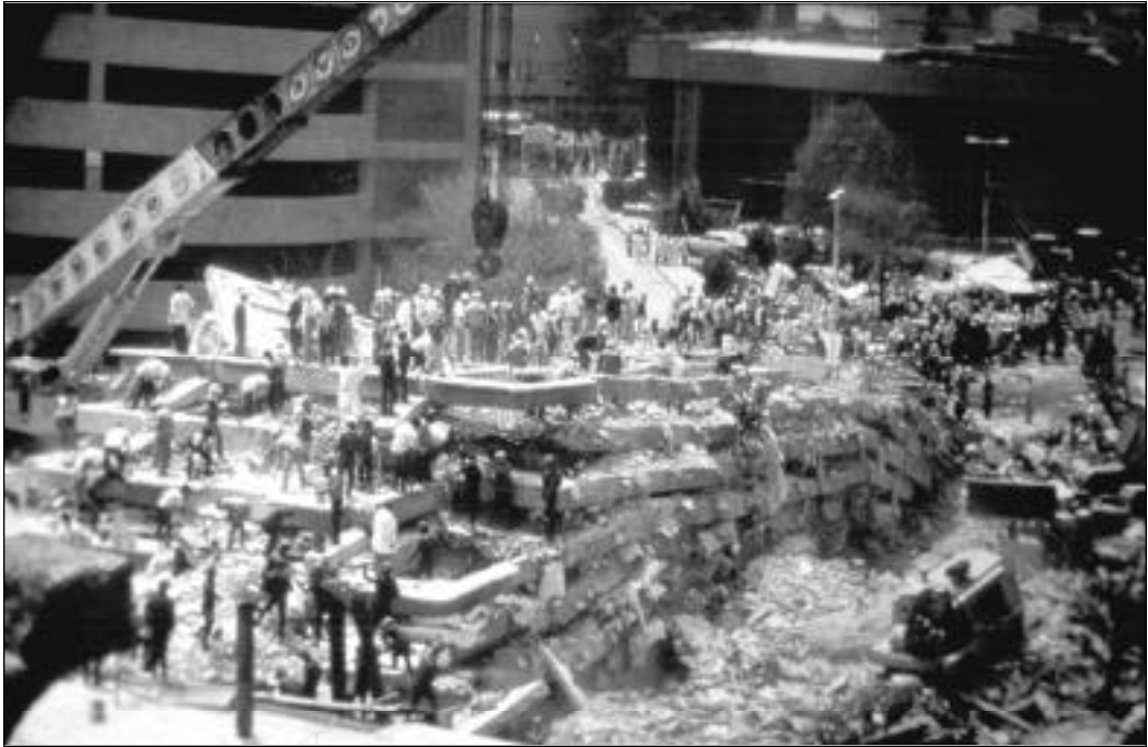
Photograph 1. Total collapse of the Benito Juárez Hospital, Mexico City, 1985.
