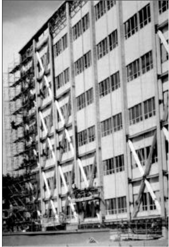
Photograph 13. Reinforcement with diagonals.
