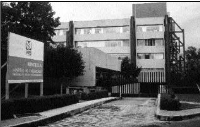
Photograph 12. The Cardiology Hospital of the Mexican Social Security Institute was retrofitted using buttresses following the 1985 Mexico City earthquake.
