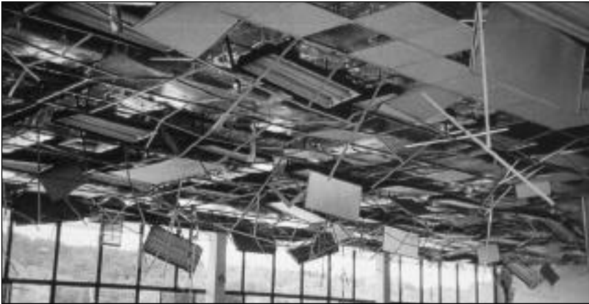
Photograph 19. Damage to ceilings
