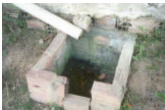
Open drainage box for household wastewater is "open house" for Culex quinquefasciatus mosquito breeding. However this box can be sealed against mosquitoes. Photo by Steven Ault, 2003.
