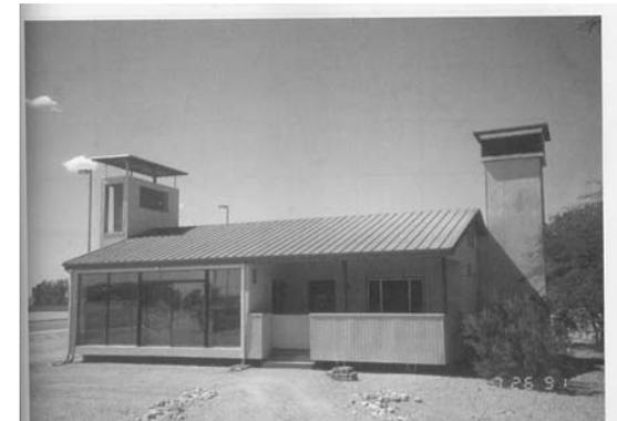
Figure S-5. The Arizona test building with the evaporative cooling solar chimney (left) and a tower (right).
