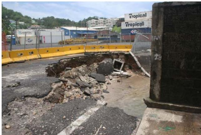
**Photo 5 – Damage to section of pavement at Shed 7**
