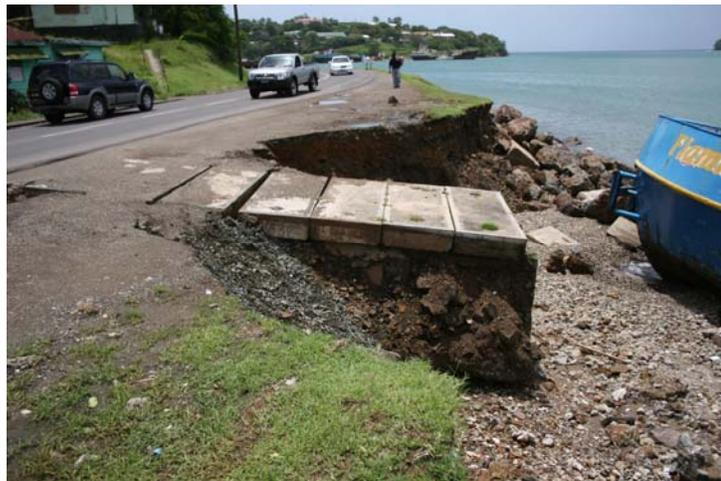
**Photo 2 – Damaged culvert and slope protection**
