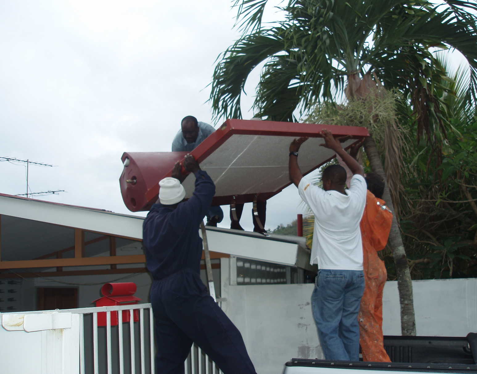
Residents install a solar water heating system on a house. Source: UNDP Trinidad and Tobago
