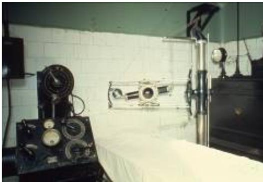
*Figure 3:* Argentina, 1965—Inadequate filtration and excessive tube housing leakage.
