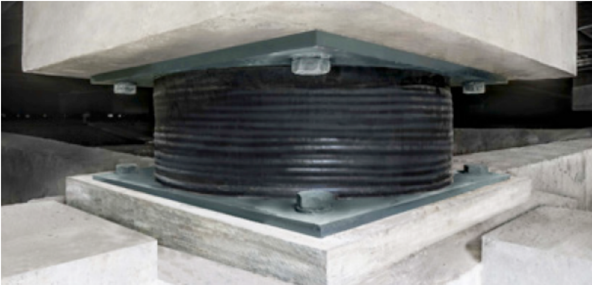
9 Photo 2 - One of the 243 elastomeric bearings (isolators), 850mm diameter supplied by MAURER
