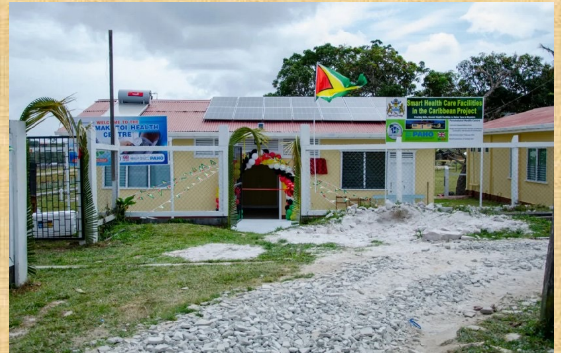
Paramakatoi Smart Health Centre Guyana
