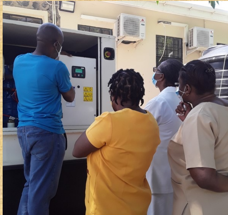
Generator training by MD Electric
