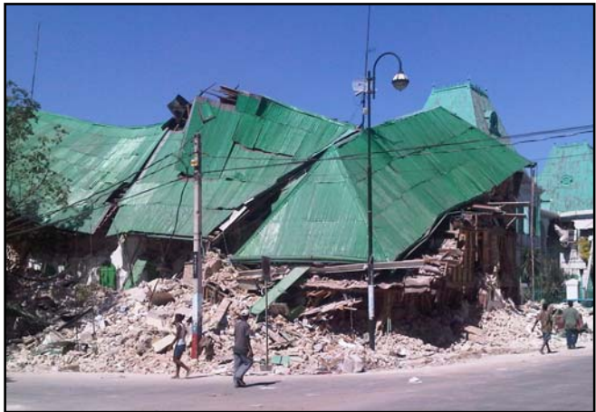
Ministry of Health Building in Haiti Photo: PAHO/WHO
